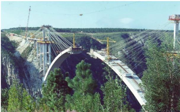
**Figure 4:** Photo showing the construction of the arch using the suspended cantilever method; Ref. [7]
