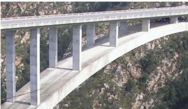
**Figure 2:** Photo showing the column, arch and deck arrangement; Ref. [1]
