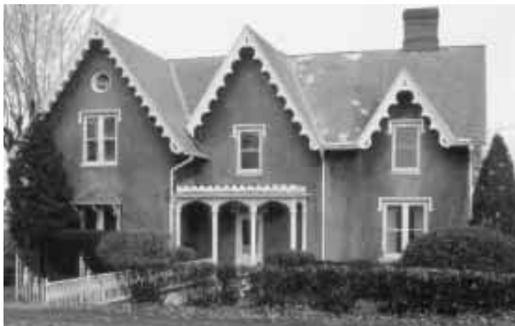
This Gothic Revival style residence in Geneva, Ontario County, New York, is typical of earthen buildings constructed in Geneva. Over 20 mud brick buildings had been constructed in Ontario County by 1855. Photo by the author.
